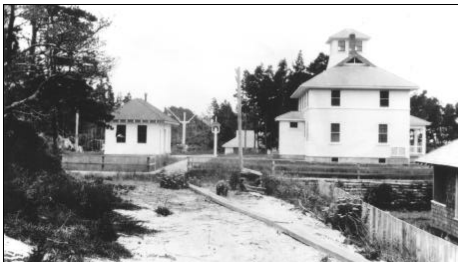
Figure 167. Siuslaw River Lifeboat Station From North, 1923. Source: U.S. Coast Guard Headquarters (Siuslaw River File).
