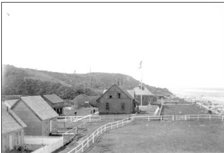
Figure 122. South Beach Station, 1904. Source: Lincoln County Historical Society (LCHS #589).
