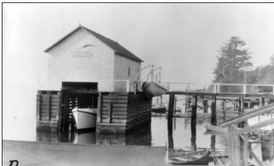
Figure 130. Yaquina Bay Boathouse, 1931. Source: U.S. Coast Guard Headquarters (Yaquina Bay File).
