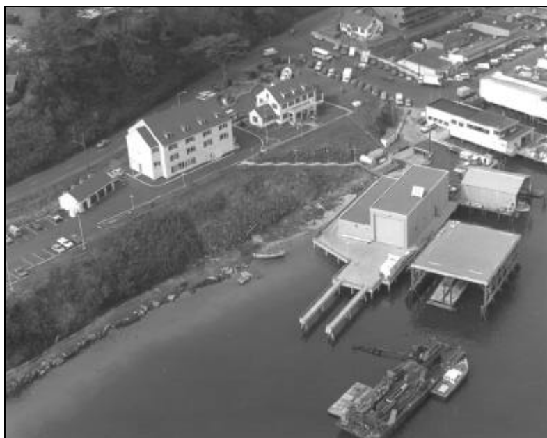
Figure 139. Yaquina Bay Station, 1983. Source: U.S. Coast Guard Headquarters (13-CGD-092283-07-06).
