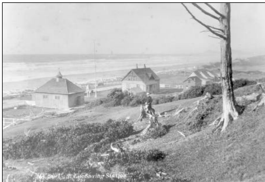
Figure 120. South Beach Station, 1906. Source: Lincoln County Historical Society (LCHS #590).
