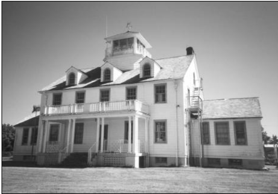
Figure 44. Point Adams Lifeboat Station (1939), Station House, in 1997. Source: Author.
