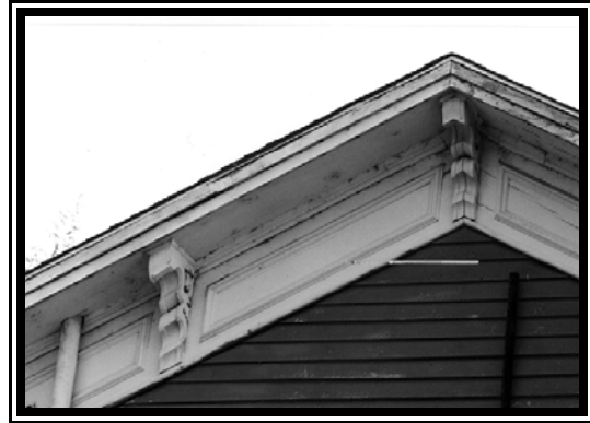
Brackets are usually constructed of several pieces and are sometimes hollow inside. The pieces can be disassembled to repair the bracket.
