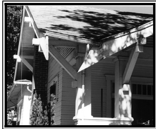
Vergeboards, projecting rafter tails, and decorative brackets are all wooden elements that might need care.
