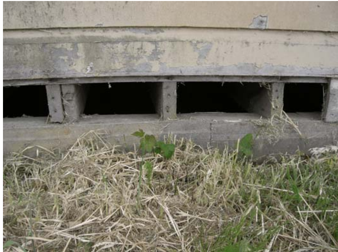
The 2x6 floor joists sitting on 4x6 beam which in turn are supported by a ring of concrete blocks.
