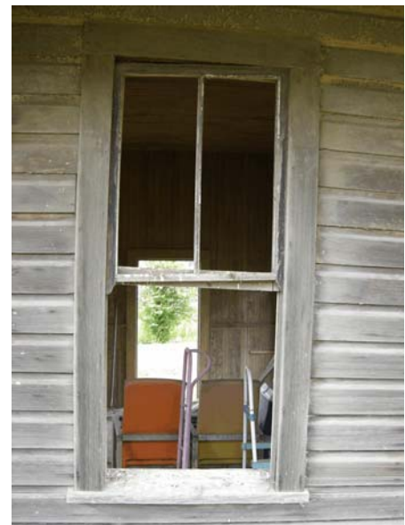
The standard 2/2 window on the south side missing a muntin.
