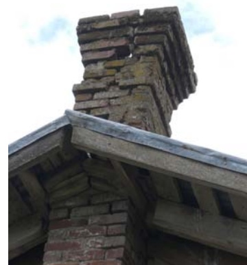
Skip sheathing at chimney.
