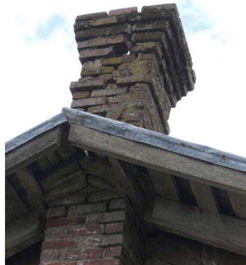
The chimney top has lost much of its mortar and is holding together only through habit.
