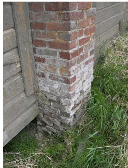
The base of the chimney has lost much of its mortar. It is unknown what is below grade.
