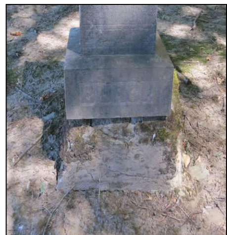
The base under the plinth of #15.25 is made of sandstone and has eroded to a dangerous degree and likely will need replacement.
