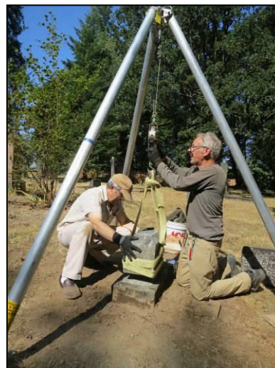
Resetting the plinth for Marker 08.19 on a bed of fresh mortar.
