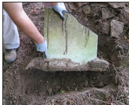
J N Flint's headstone (Marker 16.23) had been epoxied previously. The epoxy dripped out of the repaired break and then discolored over time. In addition, the stone had been reset in concrete without its original base.
