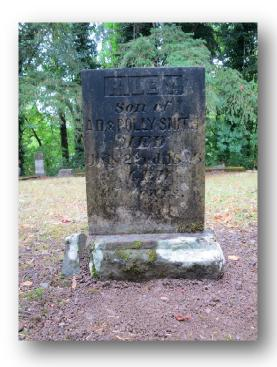
COMPLETED: Found sandstone base bedded vertically with a large spall off the north end of the base. Left spall firmly in place and leveled remaining base on bed of 3/4" minus gravel. Repaired fresh break with Akepox epoxy.
