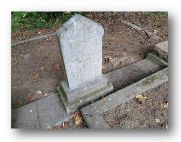
COMPLETED: Reset stone in Akepox epoxy.
