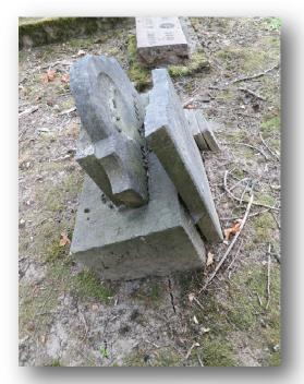
TO DO: Repair three breaks, two of which are old glue breaks.
