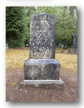
COMPLETED: Leveled base on bed of 3/4" minus gravel, reset plinth in lime mortar, and reset stone in Akepox epoxy.
