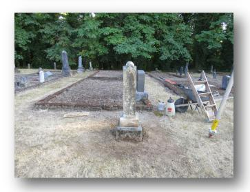
COMPLETED: Found marble footstone while leveling base and placed footstone next to base. Leveled on bed of 3/4" minus gravel, packed in, and reset stone in lime mortar.
