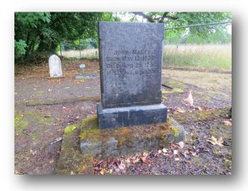
COMPLETED: Reset stone in Akepox epoxy.
