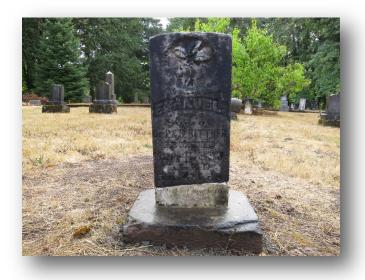
COMPLETED: Raised base 4" above grade, leveled on bed of 3/4" minus gravel, and repaired break with Akepox epoxy.
