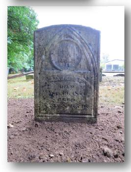
COMPLETED: Uncovered original slotted base in front of stone, determined stone bottom edge too uneven to reinsert in slot, stood stone upright at front of base on bed of 3/4" minus gravel, and packed in.
