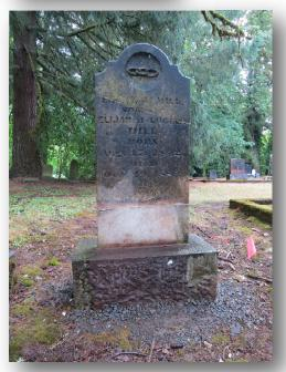
COMPLETED: Leveled base on bed of 3/4" minus gravel and repaired two breaks with Akepox epoxy.
