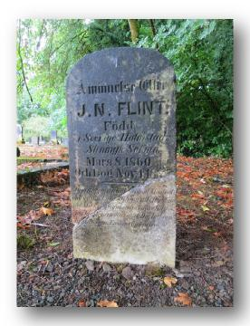
COMPLETED: Found marker bottom was embedded in concrete, so left concrete attached and leveled on bed of 3/4" minus gravel. Repaired break with Akepox epoxy.
