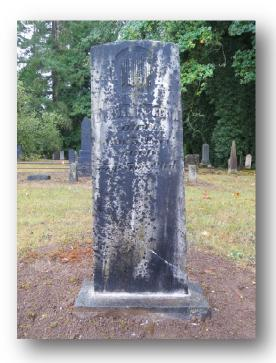
COMPLETED: Raised base 4" above grade, leveled on bed of 3/4" minus gravel, reset stone in lime mortar within base slot, and repaired break with Akepox epoxy.
