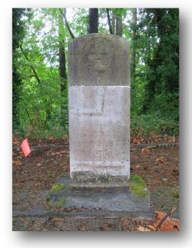
COMPLETED: Repaired three breaks with Akepox epoxy.
