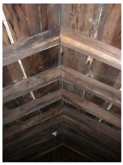
926). It has not been determined what the substance is, but if it is mold, it may have arisen from the moisture issues in this region of the roof prior to the recent repairs. Numerous mud wasp nest attachments are visible on the skip sheathing and rafters but no nests.
