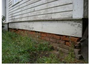
the basement window, looks to be a site drainage issue. The other, along the south elevation, is located below the wooden patch covering the foundation. It appears to be a hole dug by an animal, and it is certainly large enough for a cat or raccoon to enter. Given the uninhabited state and relative isolation of the house, this could be a concern for the short term.
