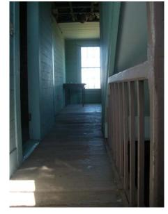
slanted edge under the stairs to the attic). The balusters are 1"  $\times$  1"  $\times$  2'3-1/8" and are spaced, from west to east, as follows: 7-3/4", 6-3/4", 7-1/8", 7-1/8", 7-1/4", 7-1/4", 7", and 10-1/2".
