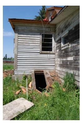
The opening at the basement window along the north elevation should be filled in before the start of the next rainy season. With regard to the south elevation hole, it should be filled in to discourage entry for small animals which could wreak their own havoc.
