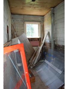
There is one door and one window in the room. The east wall contains a door next to the built-in cabinet. The door opening is trimmed in simple casing without a pediment. The window is trimmed out with the typical pediment, however, the pediment cap has been removed. The lower sash opening has also been removed and crudely filled in with modern dimensional lumber and pink insulation. The infill is as obvious on the exterior as it is on the interior.
