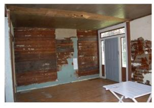
floor and ceiling along this seam and there are projecting boxed-in elements at each wall where the missing wall would attach. If the casing was removed from the projecting boxed elements, most likely a mortise for a diagonal wall brace would be seen.
