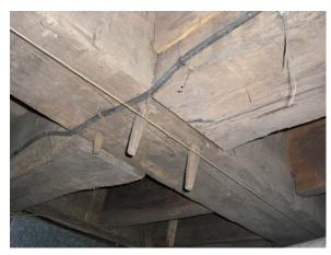
interior of the pocket. In addition, there are two beams running north-south dividing the room into thirds and acting as large floor joists. At the intersections of these beams, the connections are mortise and tenon joints with exposed treenails. At most of the intersections, the vertical heavy-timber posts intersect creating a complicated joint. Adze marks are plainly visible on the beams and on the underside of the flooring.
