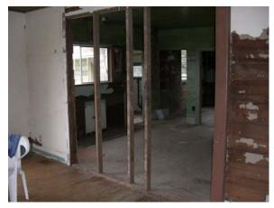
surrounded by a simple 5-1/4" plain casing rather than the formal pedimented casing of the windows. If the foyer wall had not been removed, this door would have been at the rear of the foyer. What is intriguing is that the backside of this door opening has the formal pedimented mouldings of the Center North Room.
