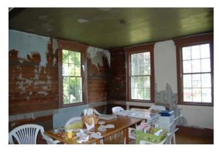
The sheathing on the walls is simple 3/4"x5-3/4" horizontal boards. These were covered in a cardboard-like cladding (1/16" thick gray paper) and then wallpapered. Most of the cardboard and wallpaper has been removed; however, there is a large remnant of the floral wallpaper on the north wall. Most likely these walls were originally covered in muslin and wallpapered.
