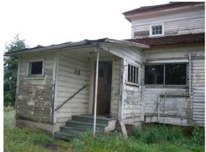
The porch now consists of an L-shaped enclosed space with covered stairs on the L's interior (east). It measures approximately 11'6" north-south and 10'4" east-west. The exact interior dimension on the north-south axis could not be determined because a toilet closet located on the southern end could not be accessed. Most recently the space was used as a laundry and bathroom. It is currently used as an entrance and for storage.
