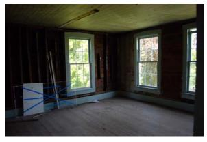
northwest room, the northeast room's floorboards run from north to south and consist of 16' long, 6-1/4" wide and 1-1/8" thick tongue and groove. There is a patch in the floor near the west wall, approximately four feet from the south wall. This may have been the location of a heat register.
