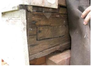
Replacement boards look to be flat grained, contain more knots, and in some cases, are rough sawn, exterior grade (west elevation). In some areas, such as along the south elevation, replacement siding has been attached with finish nails. These are inadequate to the task as evidenced by the loosening of these boards from the wall. Furthermore, replacement cladding generally
